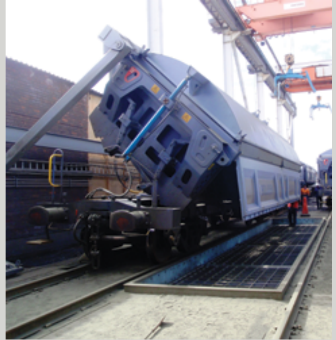
SD Unloading Station operates in the Boliden smelter in Rönnskär, Sweden.
